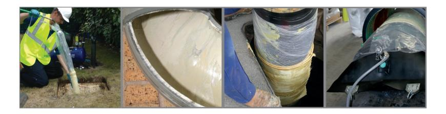
For the permanent and watertight repair of damaged pipework, without excavation.
